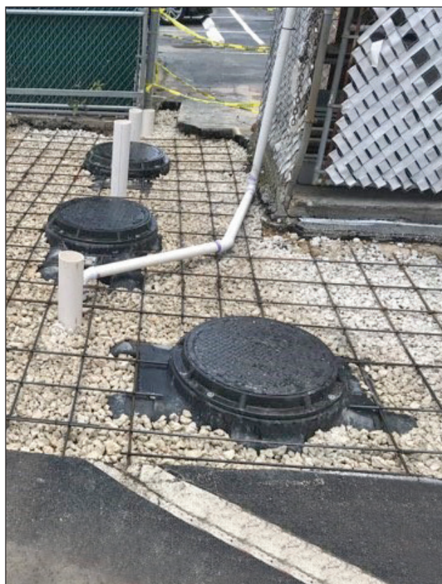
Two BIG-1150 Grease Interceptors installed in a Miami, FL restaurant
