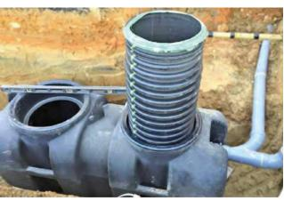
Bayer's Plumbing chose MIFAB's cut-to-fit risers for a client's grease interceptors because they make installation cost-effective and simple.
