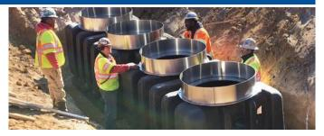
Installation Overview: MIFAB provided two SuperMax HDPE Oil Interceptors with 750 gallons of liquid holding capacity and 36" diameter custom lids for a massive public transit project called Purple Line in Landover, MD.
