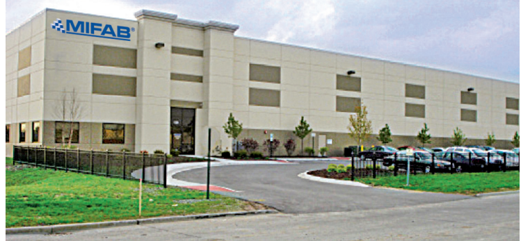
MIFAB's factory in Chicago, Illinois
